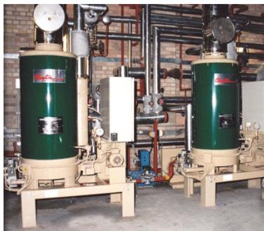
feedwater pump and the steam/water mixture which is produced at the outlet of the coil is directed to a high efficiency vortex separator. The steam quality at the outlet of the separator is at least 99.5% dry saturated.
