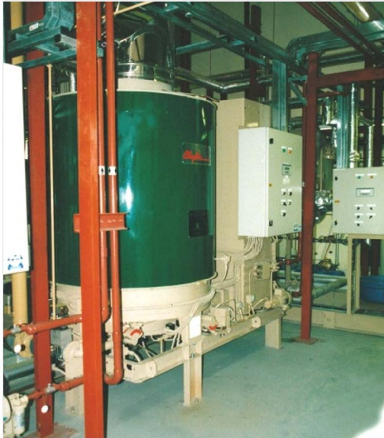
circulation monotube coil concept it is not necessary to contain large volumes of water within a Clayton Steam Generator. This produces a number of significant advantages in terms of reduced running costs, fast reaction time, size, weight and safety.
