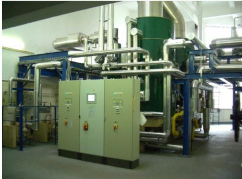
continuous helical coil in the steam generator at a controlled rate from the top of the coil to the bottom. At the same time the hot combustion gases from the bottom mounted burner pass heat upwards over the coil in the opposite direction.
