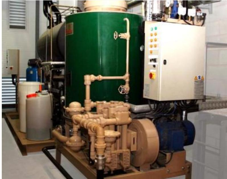
Clayton Steam Generator is one of the vital parts of this bread making process where steam is essential in the retort cycle for sterilization of the finished
