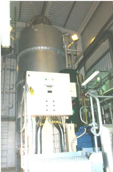
The driving force behind the project was the commitment of Medway Power Station to 'flexible operations' which involves the plant being shut down and re-started, as required, in response to electricity demand and prices. The new Clayton steam generator allows the station to be brought on-line and achieve base load significantly sooner after a
