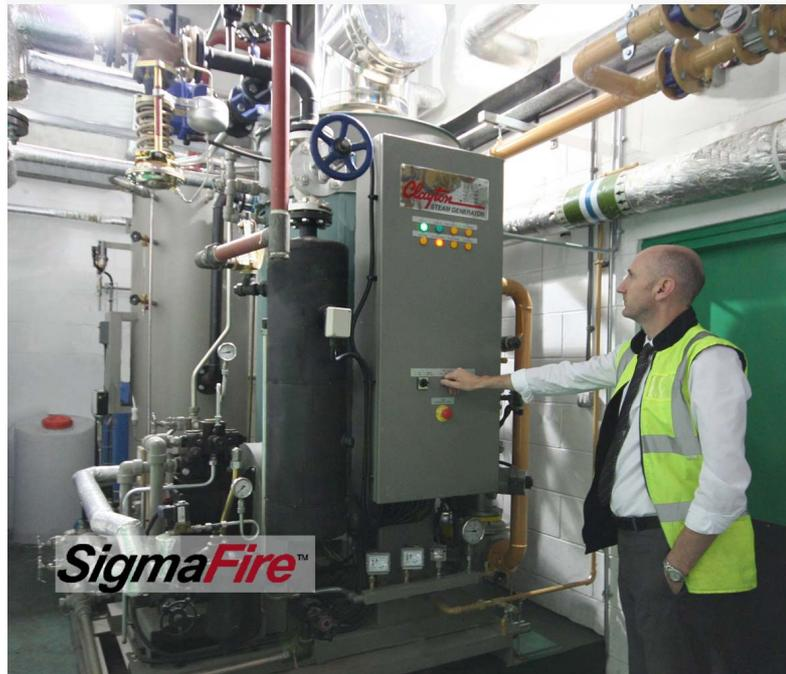
**SigmaFire Clayton Steam Generator** that provides steam as the heating medium for a new high quality fresh pasta line.
